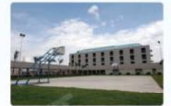
Dormitory and recreational facilities
